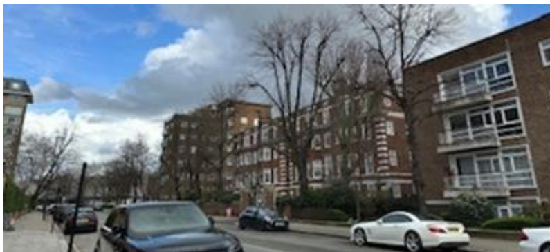
Photo 3: Mancroft and neighbouring residential buildings to the north of the site
