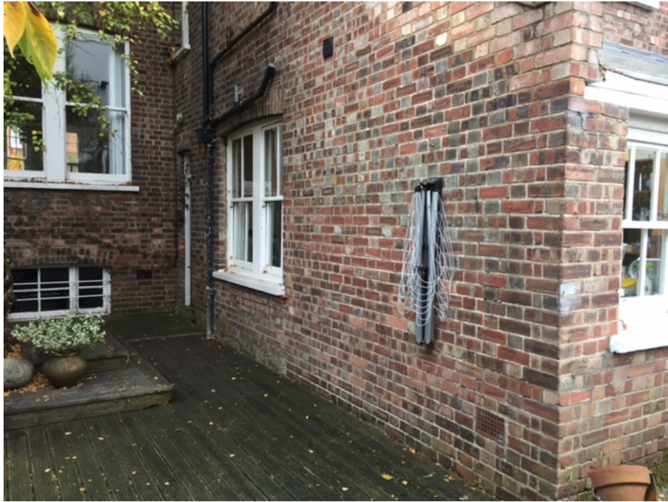
Photo 3: side elevation of rear closet wing
