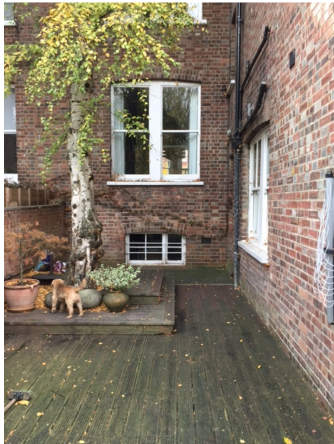
Photo 2: Existing rear elevation
