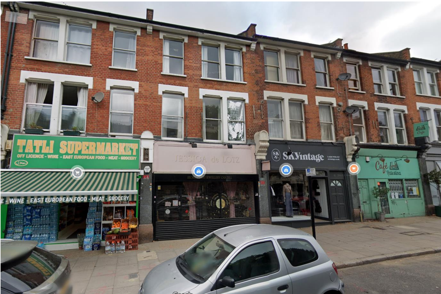
Figure 4: Existing retail units on Fortress Road (to remain), note: no changes proposed to street elevation.
