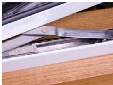
Restrictor hinge for child safety
