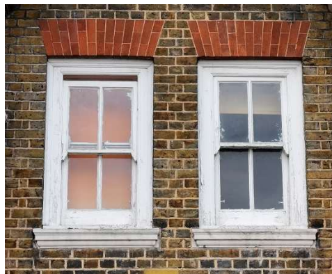
Figures 2 and 3: Visible deterioration to timber windows
