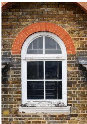
Figures 2 and 3: Visible deterioration to timber windows
