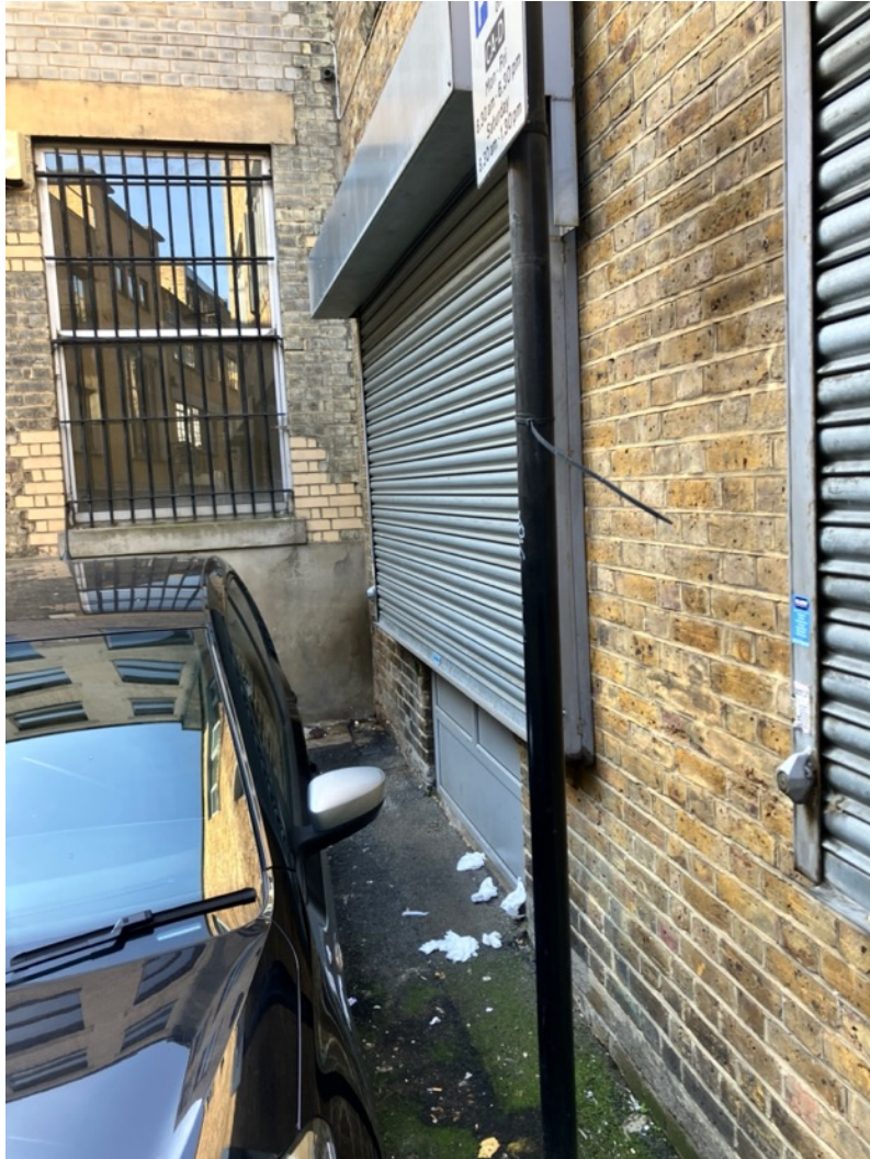
Fig 3. Detail of existing roller shutter with former door opening visible. Evidence of anti-social behaviour, with human waste and toilet tissues present.
