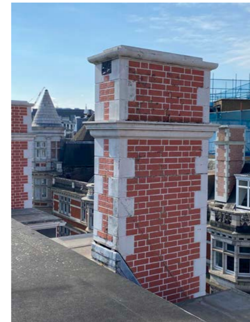
1980's replacement GRP chimneys
