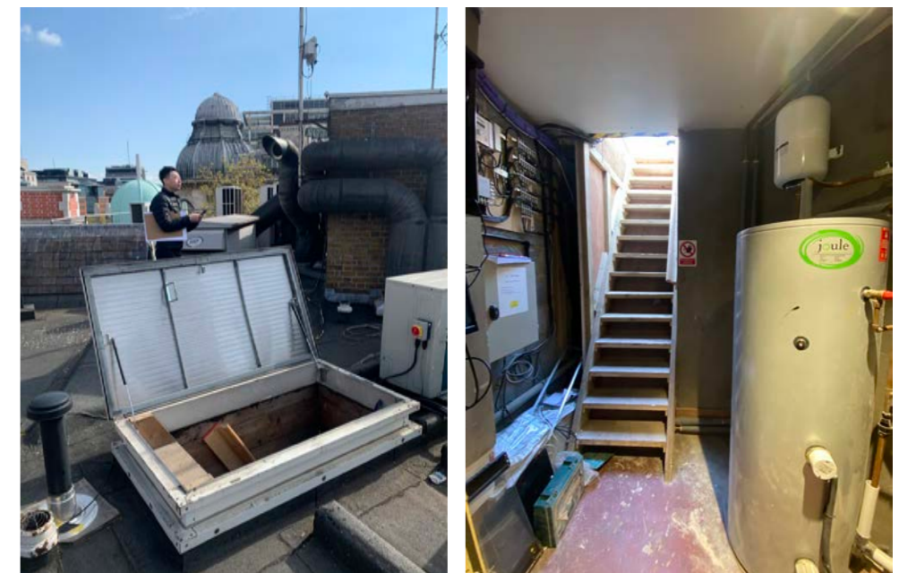
Current access steps to roof level
