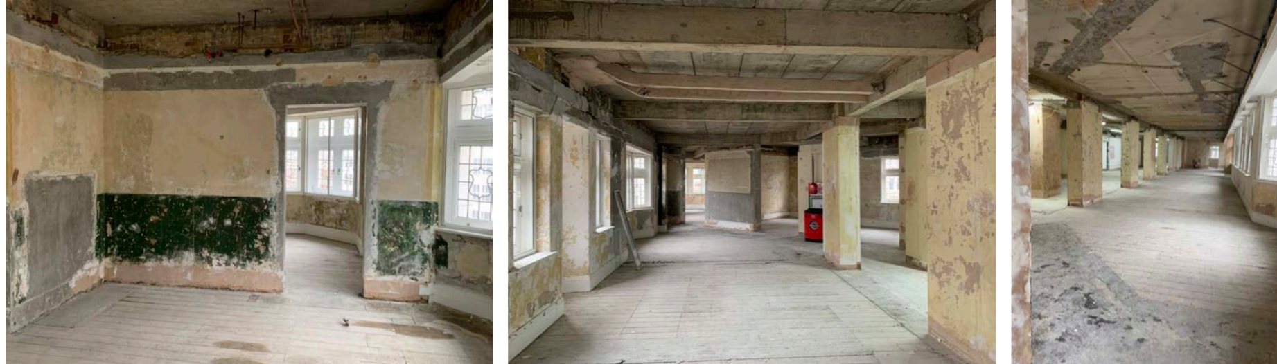
Office floors post-strip out works
