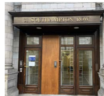
Current shared entrance with recessed doors and projecting canopy
