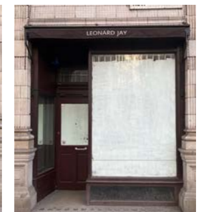
Awning box projects over the doorway incorporating modern door.
