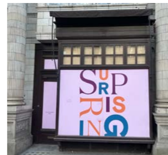
Awning box sits higher than others. Openable high level windows.
