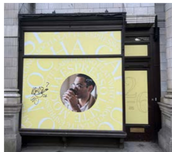
Awning box does not project over the doorway. No high level vents.
