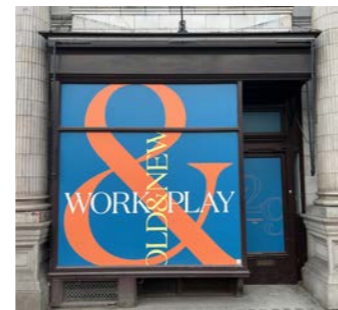
Modern shopfront with extended awning box
