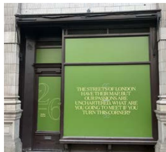
Awning box extended to project over the doorway. High level vents retained
