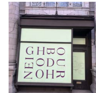
Modern shopfront with extended awning box
