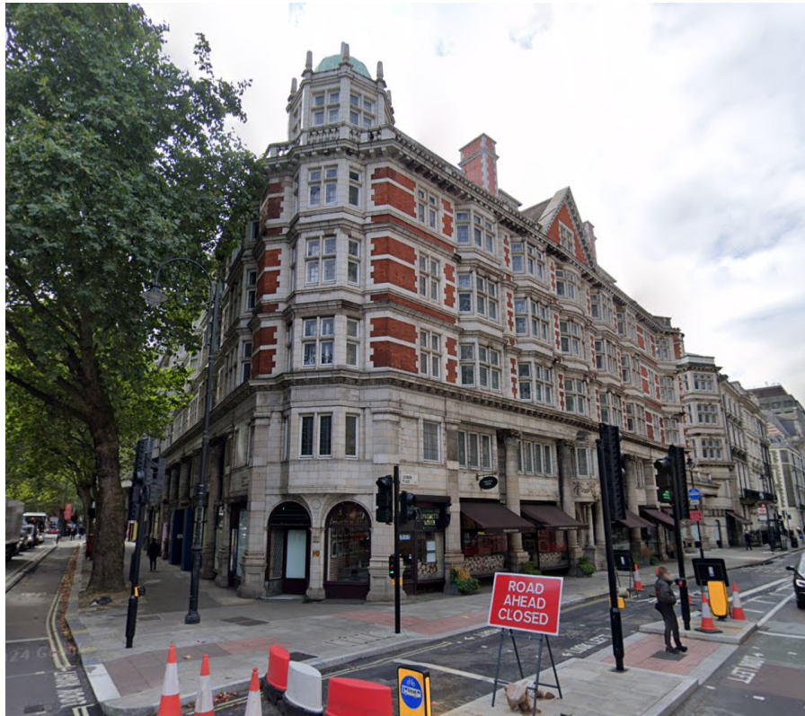
Figure 1: Existing building at 31 Southampton Row
