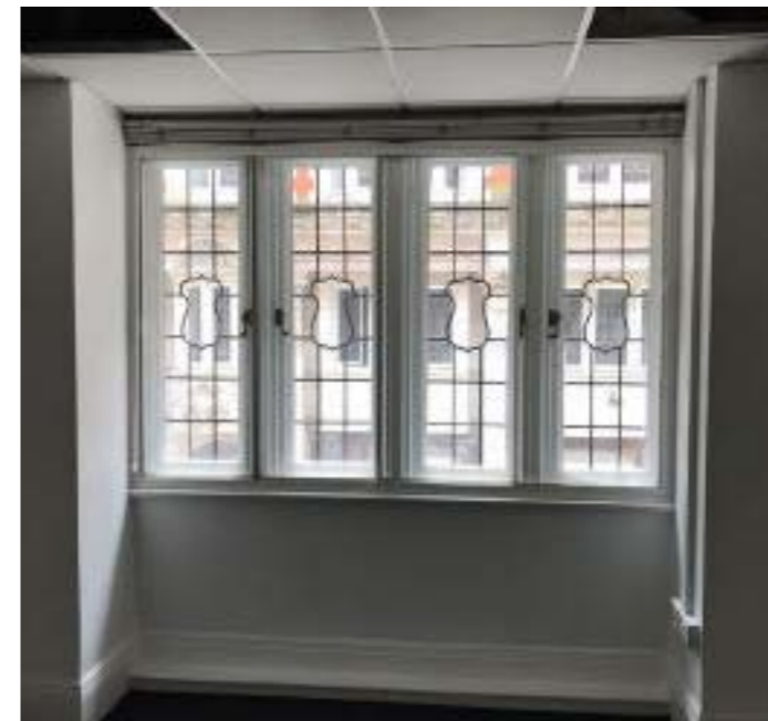
Figure 4.7 Original windows sat behind secondary glazing
