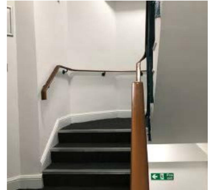
Figure 4.4 Modern stair located in historic lightwell
