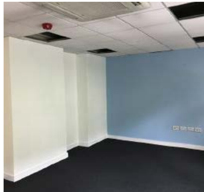
Figure 4.6 Office on second floor level, but typical of office space within the building
