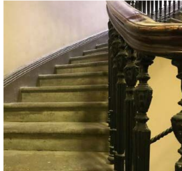
Figure 4.2 Historic primary staircase
