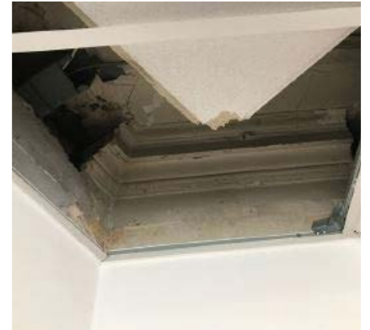
Figure 4.8 Historic cornice present beneath suspended ceiling
