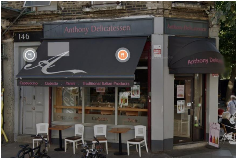
1. Existing front elevation photograph from GoogleMap
