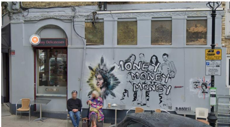
2. Existing side elevation photograph (Sharples Hall Street) from GoogleMap
