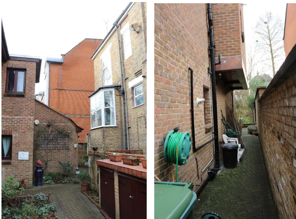
Figures 6, 7. View of the front and side passage to be infilled.
