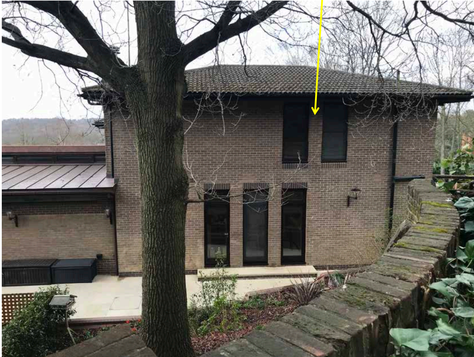
PHOTO E - Residential property, in Highfields Grove, over the boundary wall at the bottom of the back garden
