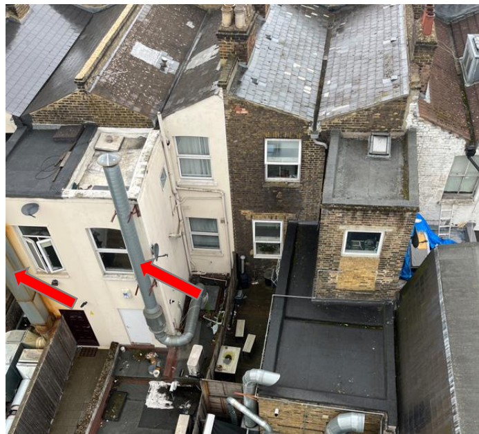
Figure 4 – Flues and plant equipment of Papa Johns and KFC (red arrows), Nos 53 - 55.
