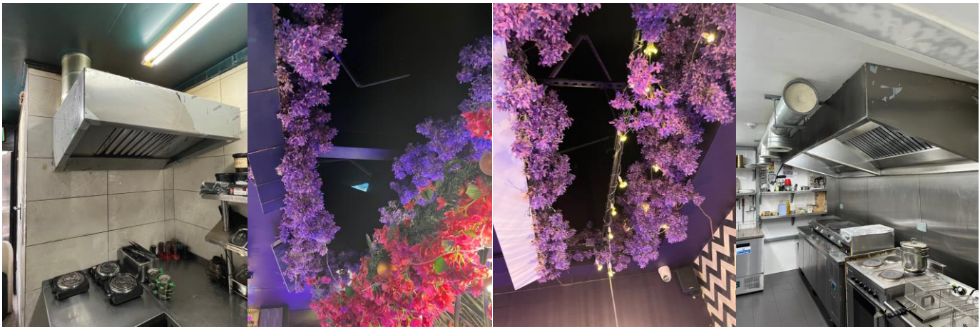
[LEFT] – Extraction fan connecting to the flue at the rear of No 49 (coal fumes)
