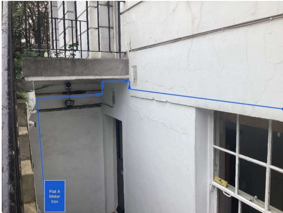
Figure 1 Proposed pipework to basement lightwell.
