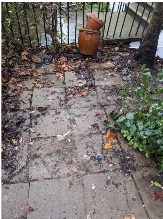
Existing pavers – damaged in need of replacement
