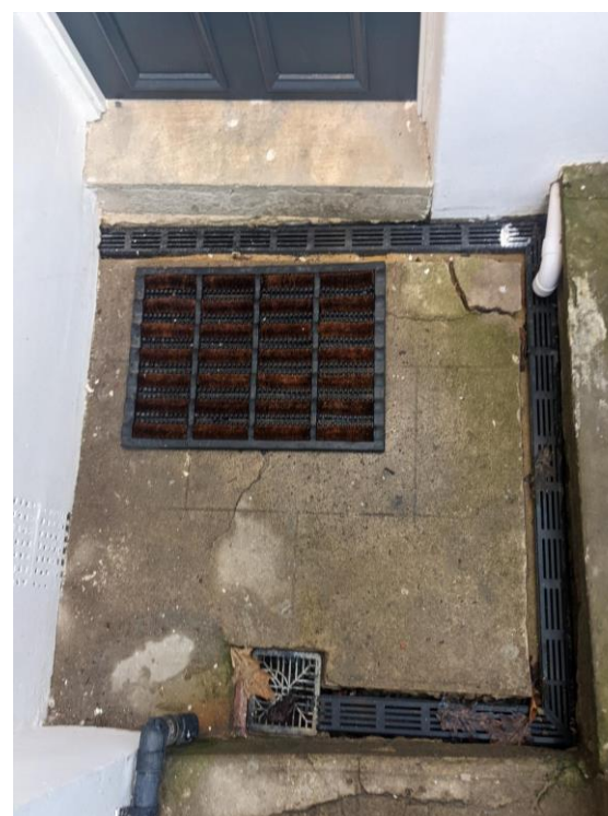
Existing footwell drain with linear drain surround
