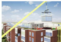
3. Module Installation (Note: design indicative only).
