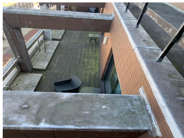
Figure 6: Existing materials comprise brown brick and brown tiles. Parapet and arches have lead flashing
