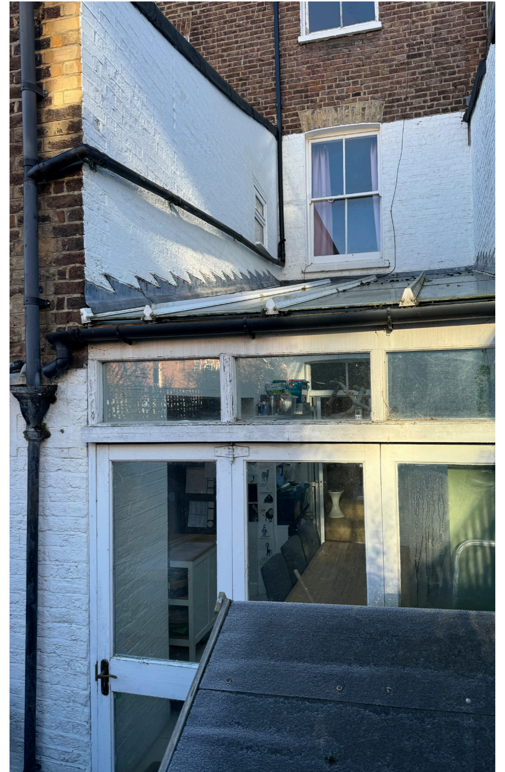
South-West (Closet Wing Flank) Elevation
