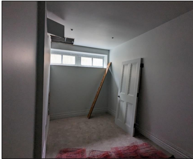
Figure 4.14: Visual clues of the garage door visible from inside the mews building
