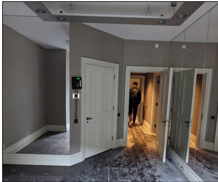
Figure 4.9: Rear room at basement level
