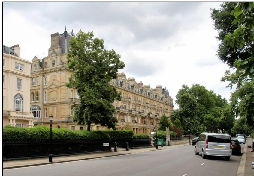
Figure 4.1: View of Cambridge Gate taken from the North
