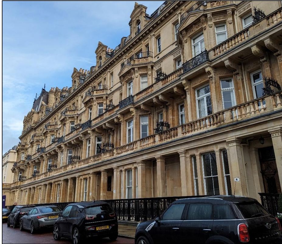
Figure 4.17: Photograph of Nos. 1-10 Cambridge Gate
