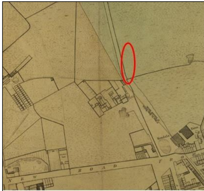
Figure 3.1: An Extract from Richard Horwood's Map of London (1799), with the approximate location of Cambridge Gate circled in red.
