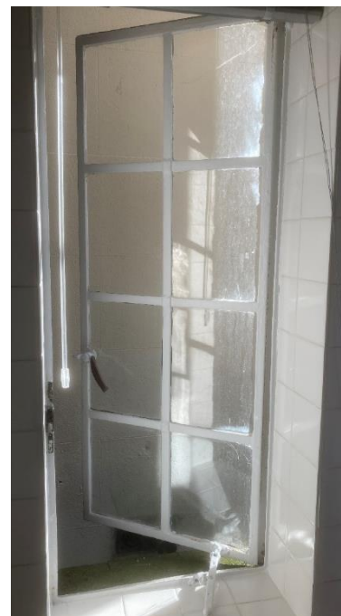
Figure 4a – Existing Window
