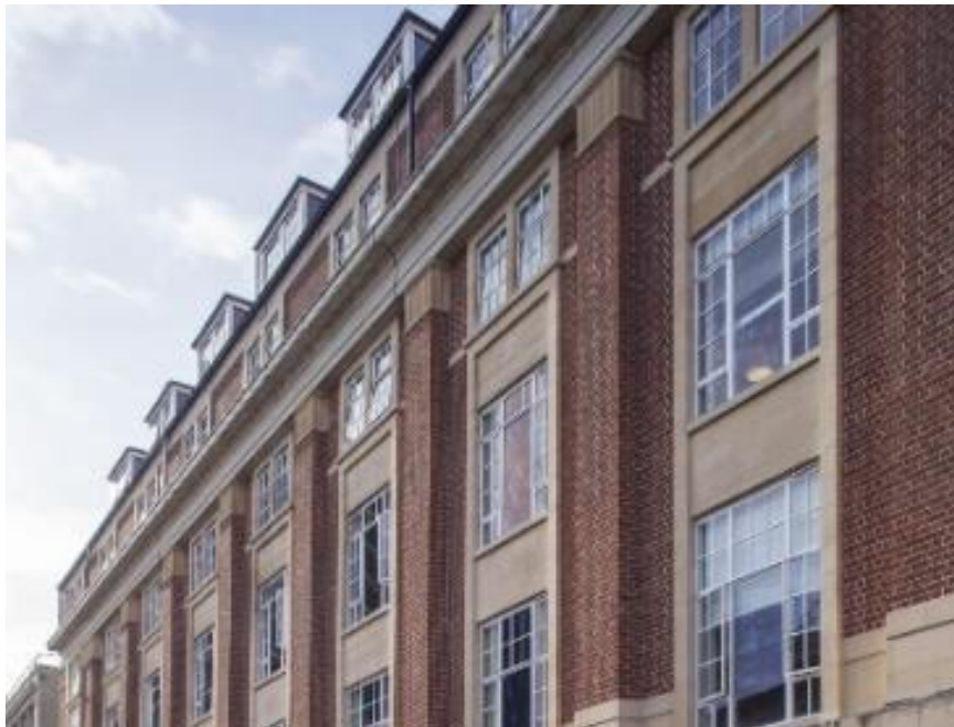
Figure 10c – Installed Alitherm Heritage Windows at Colston Street, Bristol (front elevation)
