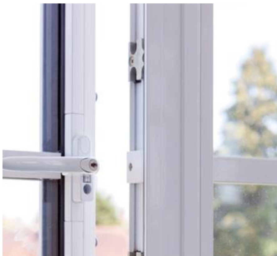
Figure 8 – Windows at Lanchester Free School
