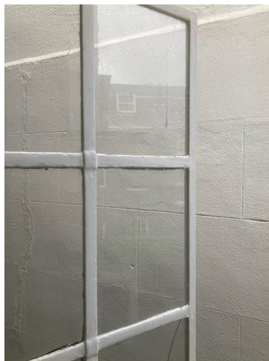
Figure 4b – Glazing bars - Internal
