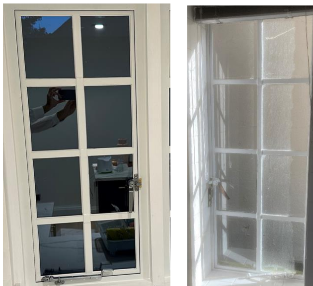
Figure 17b – Design Alternative 2 – Glazing Bar Pictures
