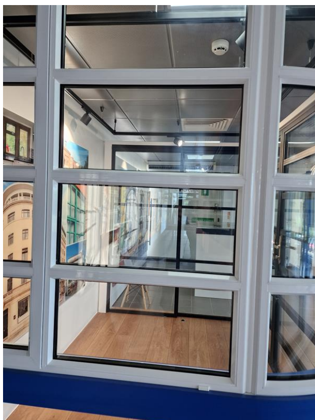
Picture of transom-style fixed glazing bars
