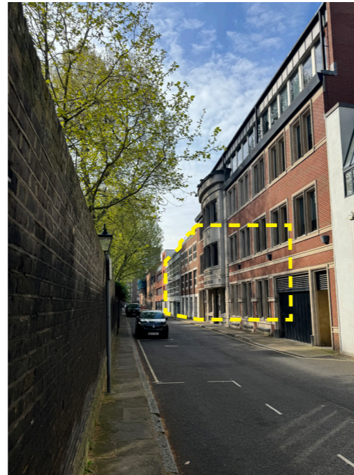
A - Long View looking South - Existing Roofline
