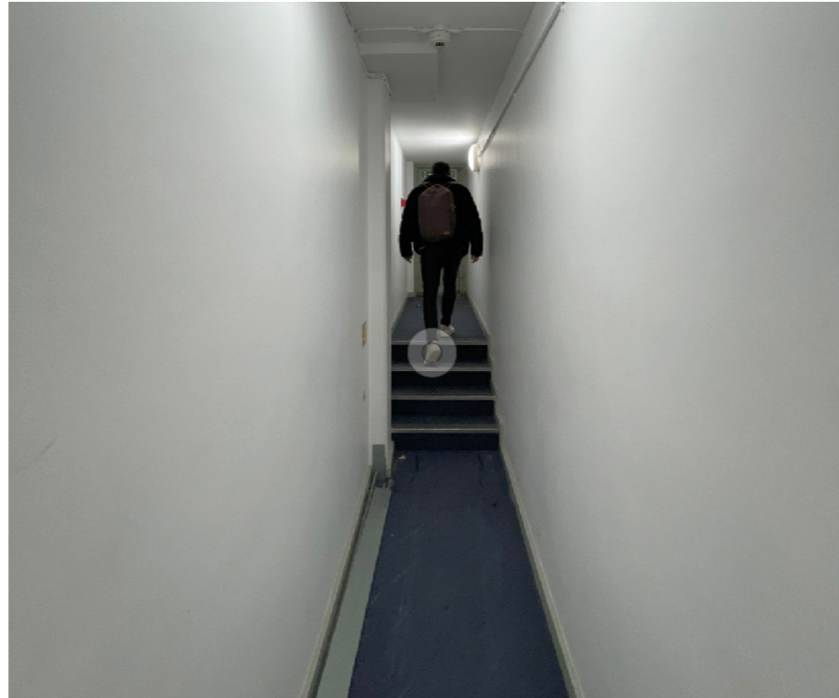
Restricted fire escape route to Jockey's Fields
