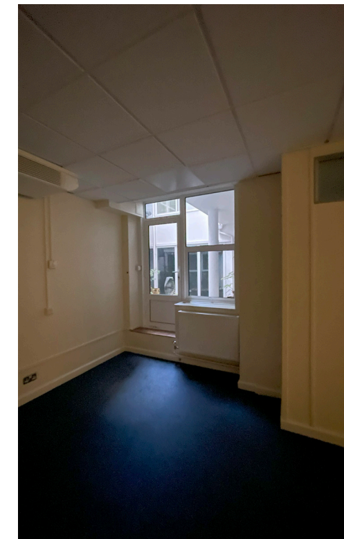
Access to existing lightwell
