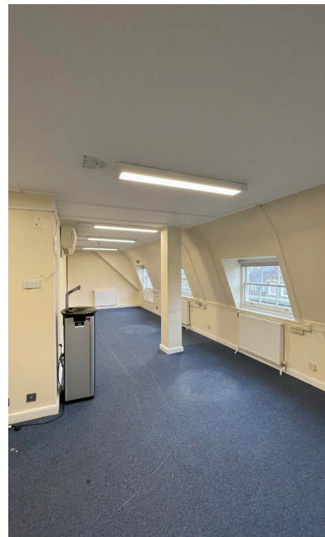
Level 04 mansard room
