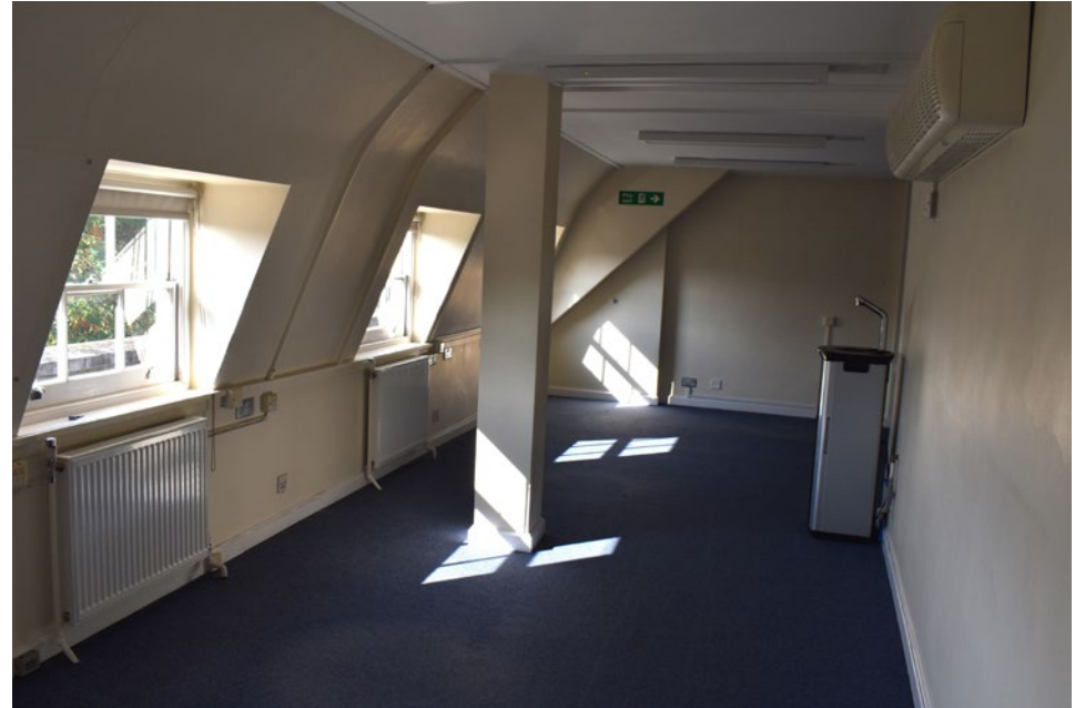
3.16 14 Bedford Row, dormer windows in the fourth floor front elevation
