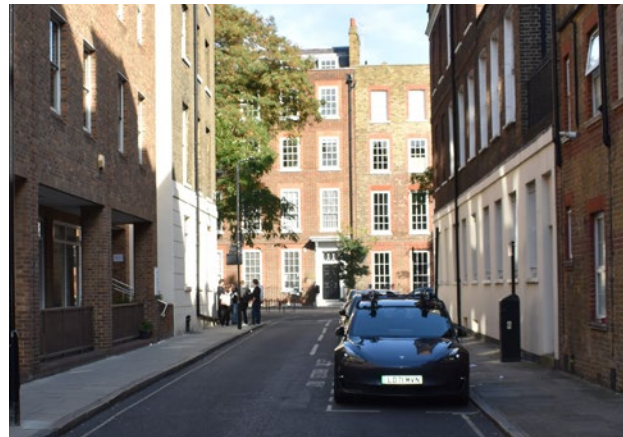
3.2 Numbers 13 and 14 Bedford Row seen from Princeton Street. The mansard floor was added to Number 14 in 1981
