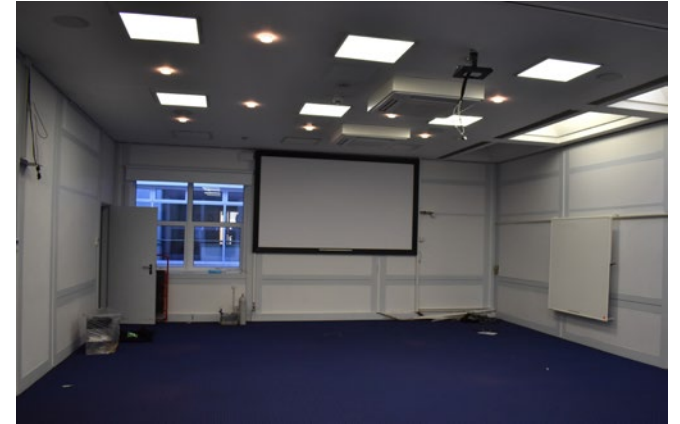
3.21 Link building, upper level
