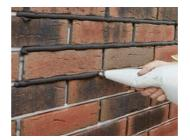
**3.** Specially formulated mortar is then piped into the brick joints.
