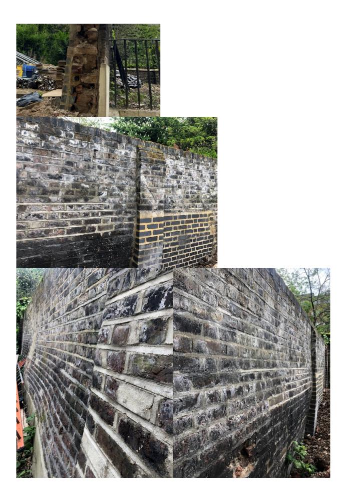
The wall is bowing and there is a large crack running between the internal masonry and external leaf. The wall appears to be unstable and unsafe to be maintained during underpinning works. It is our recommendation to demolish the wall the full extent to allow the retaining wall works to be carried out.
