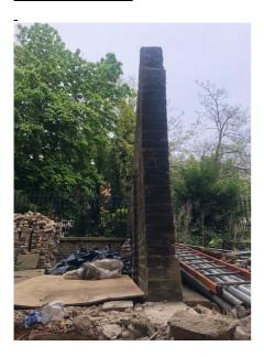
The wall has a significant lean and we have concerns with the walls stability during underpinning works. It is our recommendation to demolish the wall the extent of the currently proposed underpinning works, to allow the retaining wall works to be carried out. Attached are the current underpinning works and foundation plan for reference.
