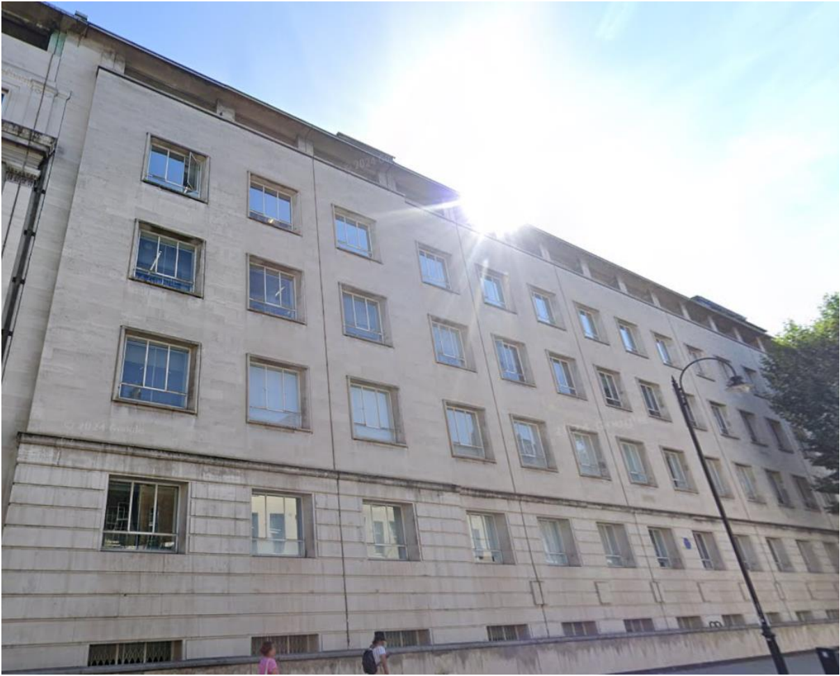
1. Street View image of the building from Gower Street
