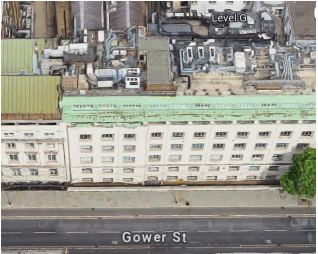
2. Aerial image showing the roof and existing plant units
