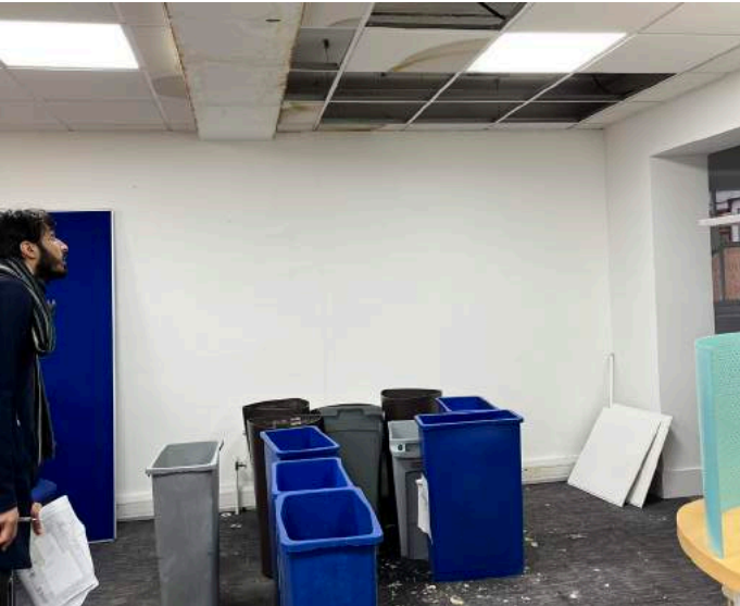
5. Block G roof leaks
