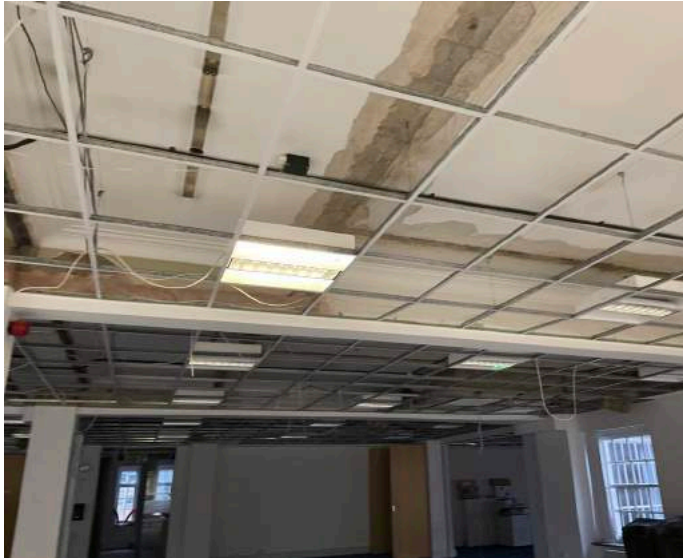
2. Block F exposed soffit visible through the stripped out grid ceiling
