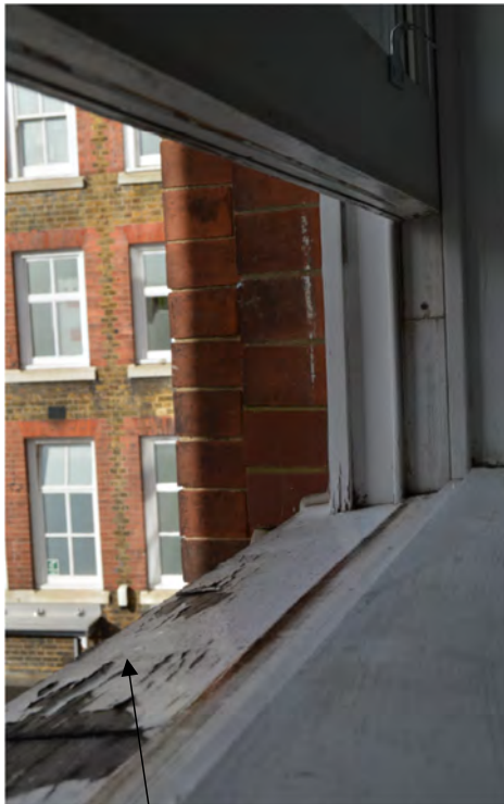
Cill failure to window when scarf repair has failed in South West Elevation
