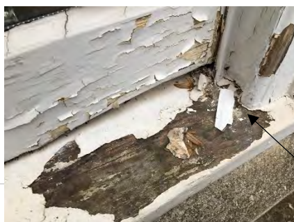
Base cill failure to window in South Gable Elevation
