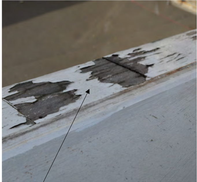
Detail of cill failure
