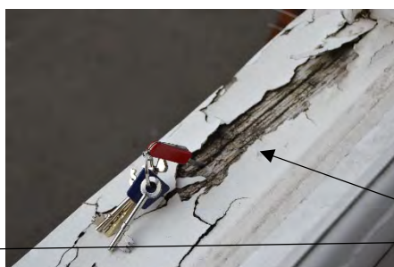
Base cill failure to window in South Gable Elevation
