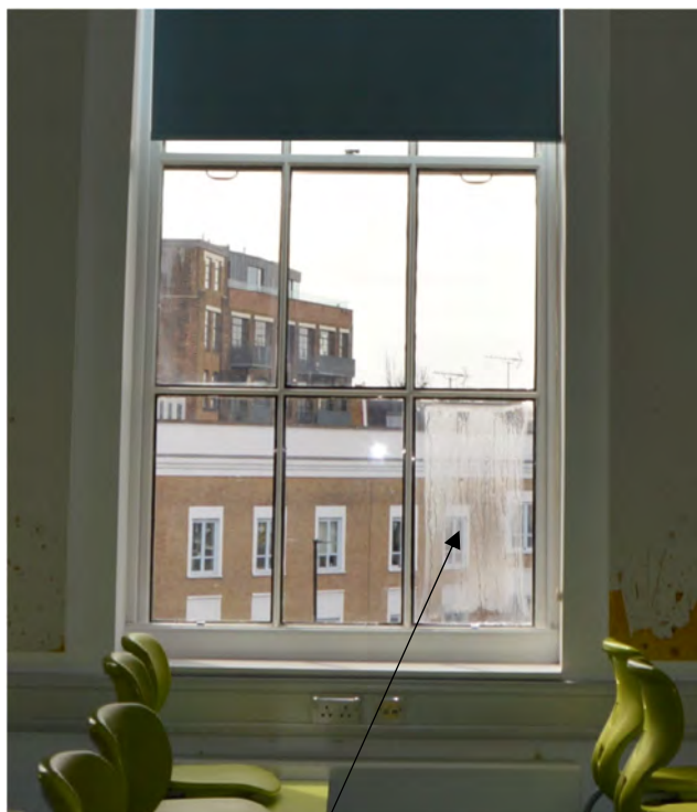
Failed Double Glazed sash to be replaced to South West Elevation
