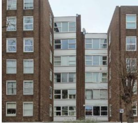
Figure 10 Continuous Vertical Panels
