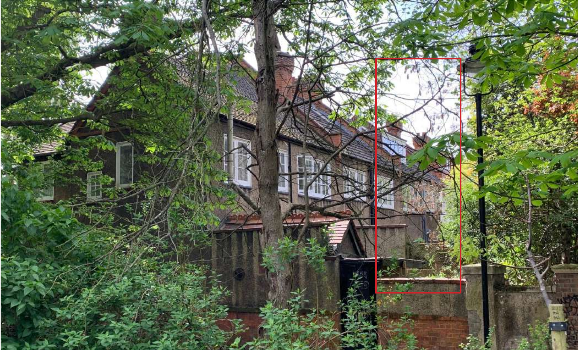
View to the rear of Glenhurst Avenue from the tree filled green space between the end of the road and Highgate Road.
