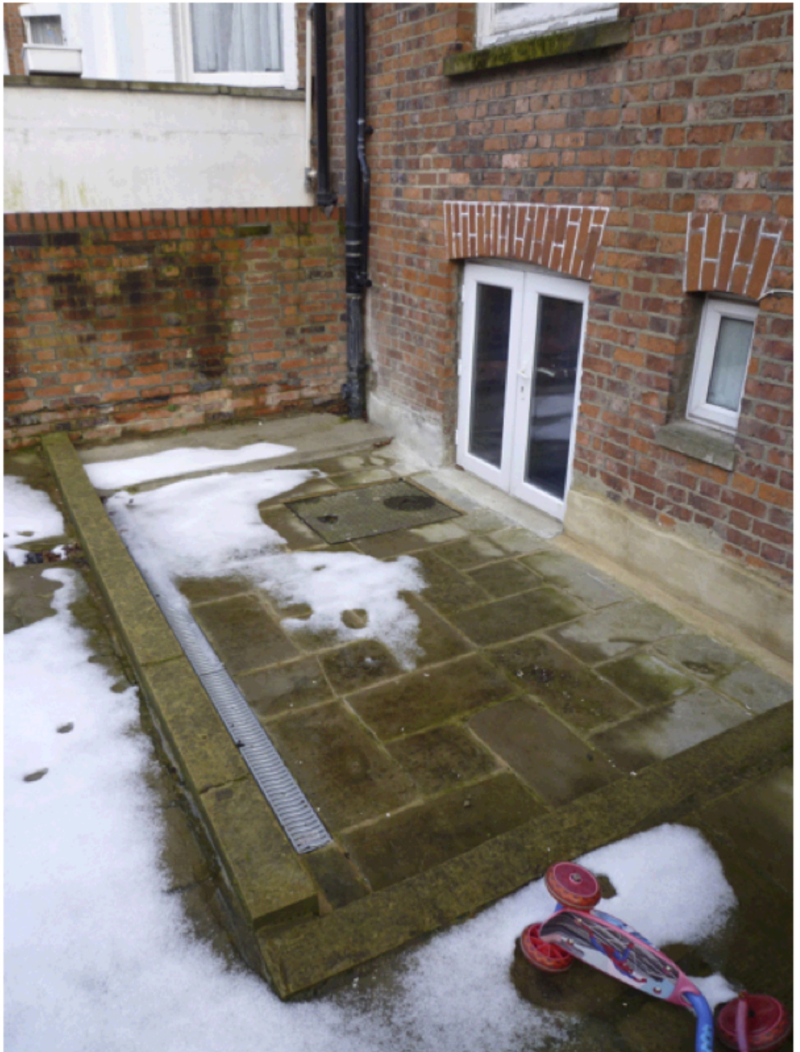
Figure 2. Photograph of the rear windows to the existing basement.
