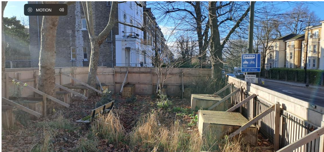
Photo 2 of T9 – T14 looking showing internal struts and above ground stillages
