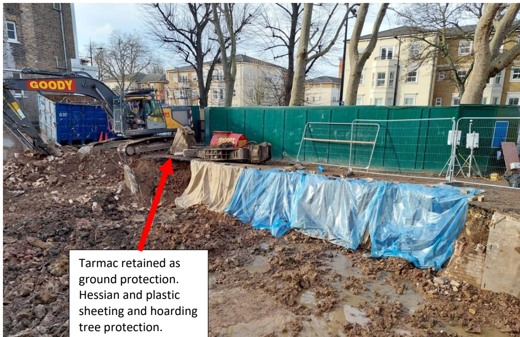
Photo 1 of the completed demolition
