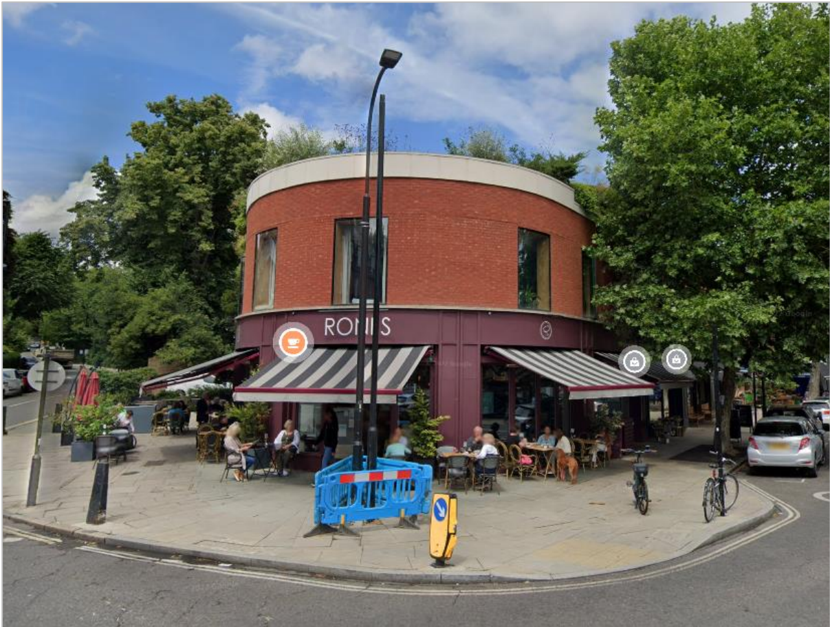
Figure 1: Google Street View Image of the application site (dated June 2022). Note the seating to the front of the building which brings activity, vibrancy and interest to the street.
