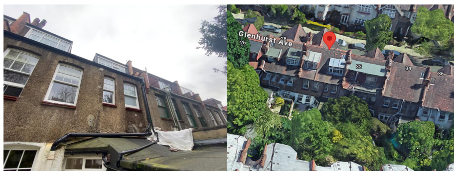
Images of existing balcony at no. 32.
