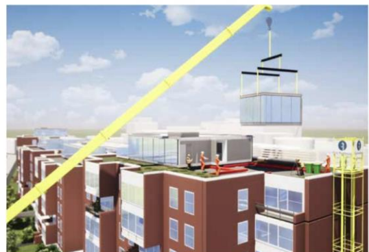
3. Module Installation (Note: design indicative only).
