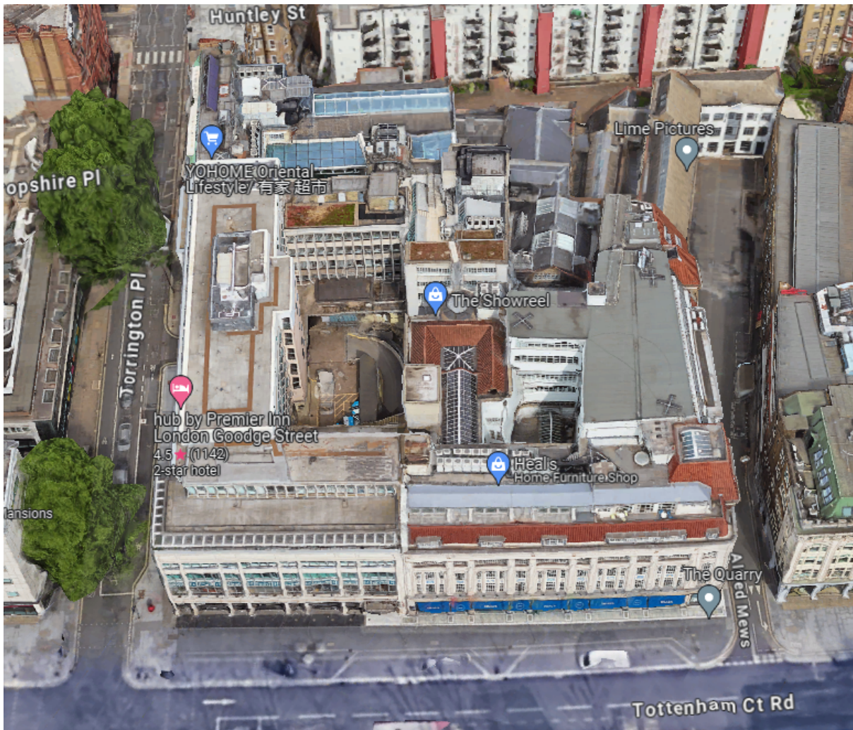
1. Aerial view of the Heal's Building
