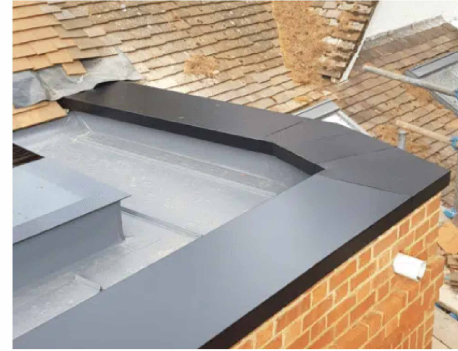
Powder coated aluminium coping 300 x 60 mm https://kladworx.com/products-and-services/aluminium-coping/
