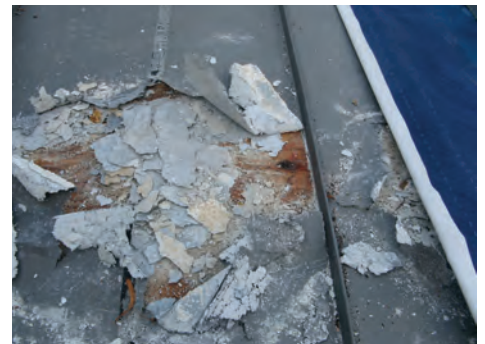
Result of using a hybrid roof.
