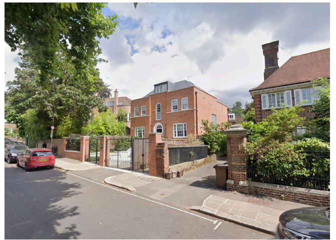
1. View from the street, the condenser is not visible from outside the property.
