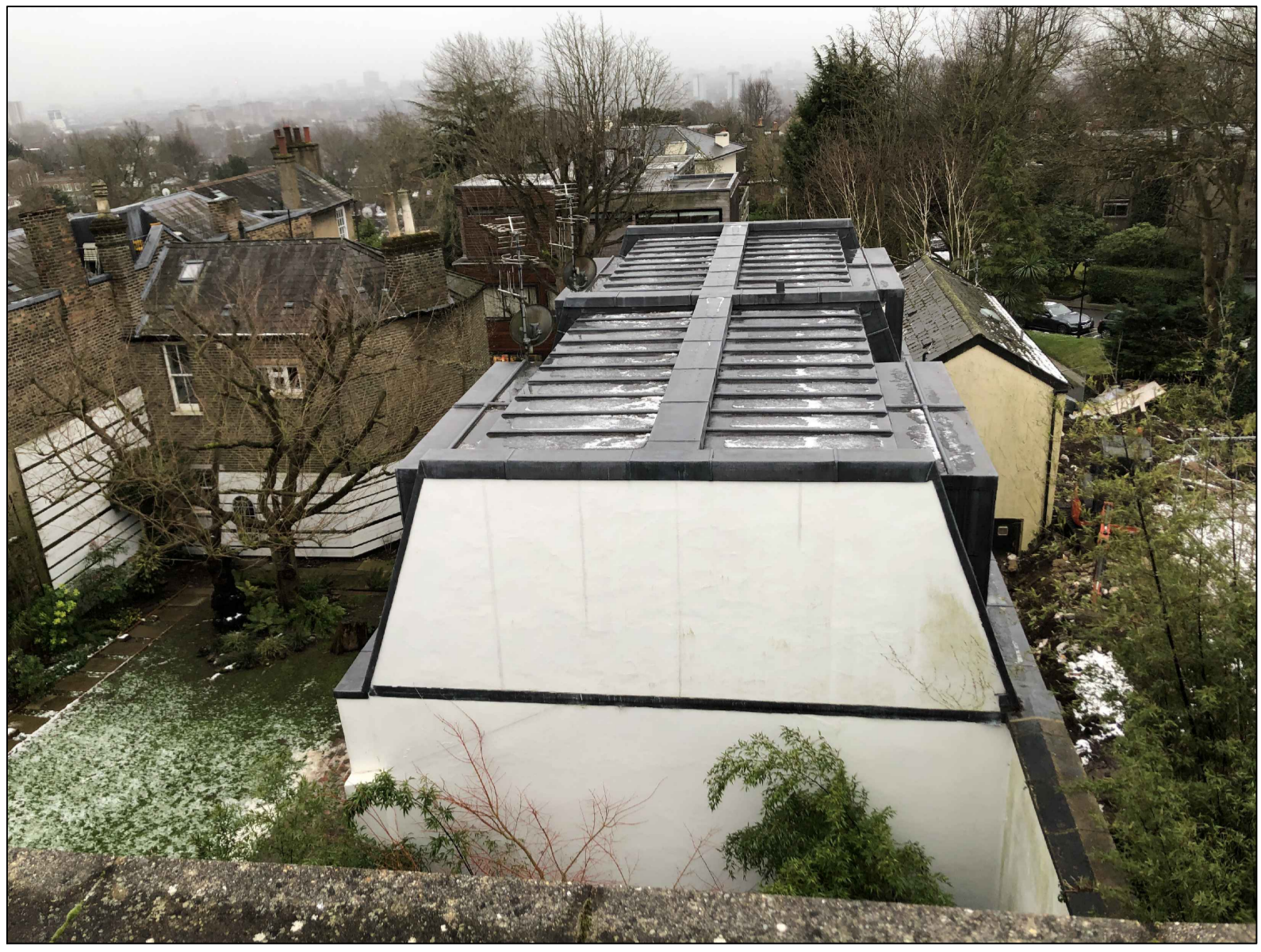
3 VIEW FROM ROOF LOOKING SOUTH NTS
