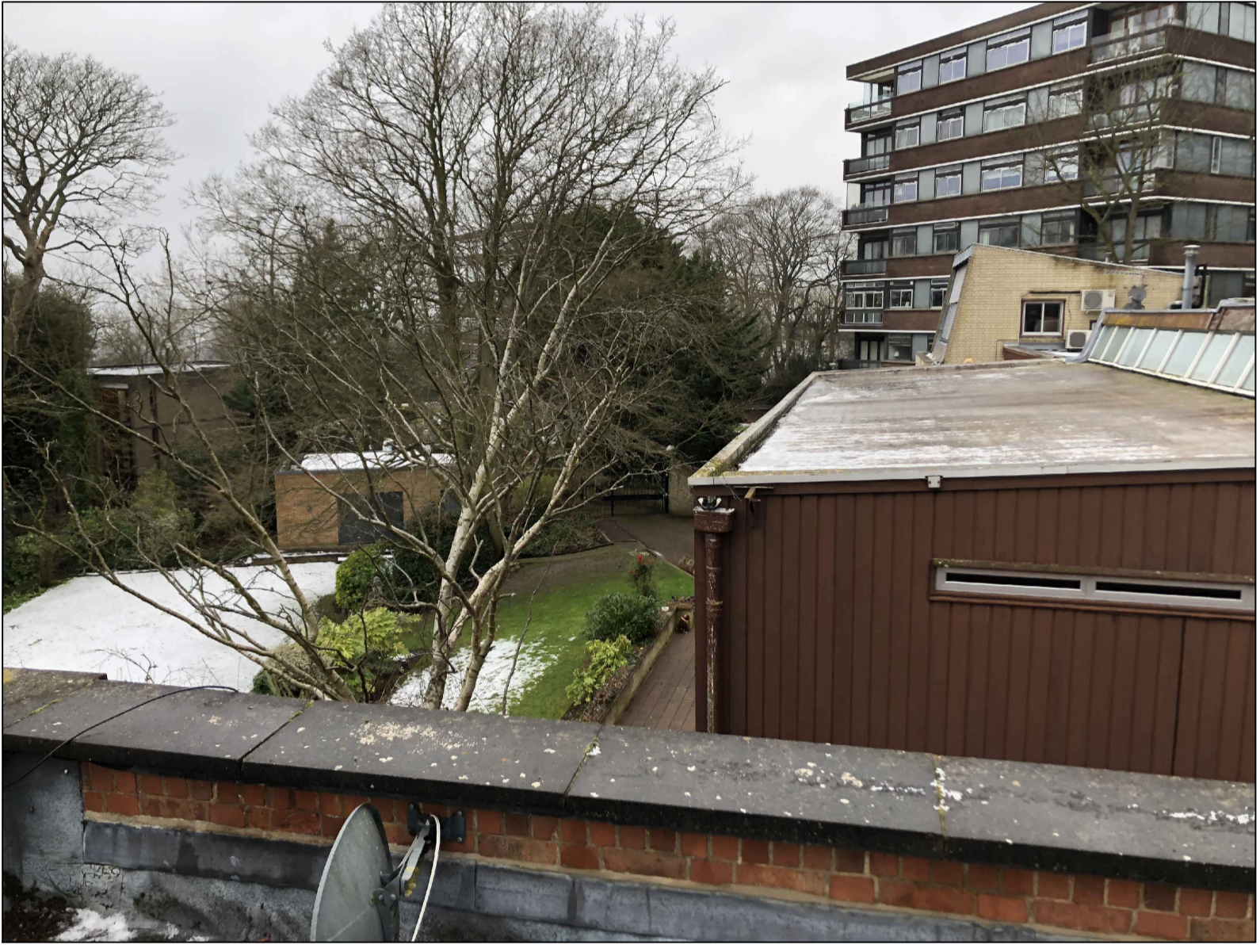
4 VIEW FROM ROOF LOOKING SOUTHWEST NTS
