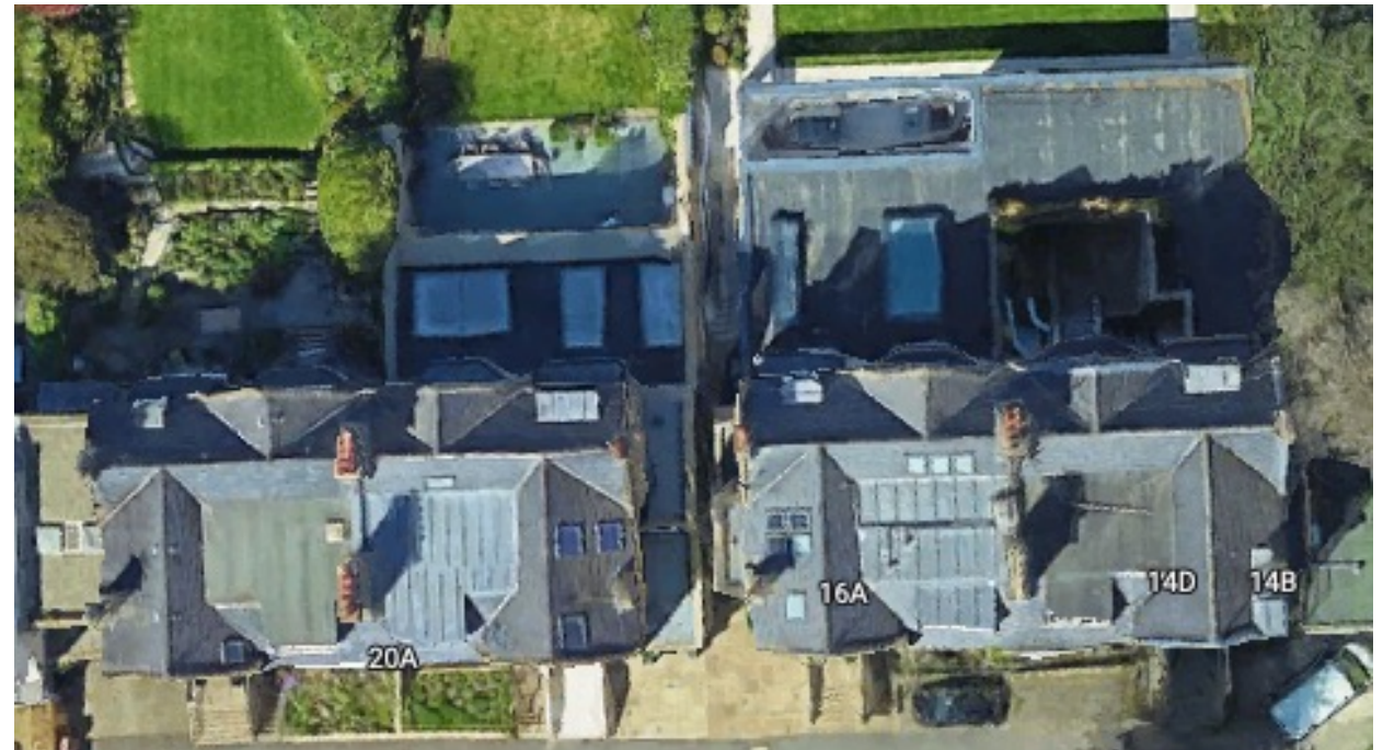
Large modern extensions built to 14 & 16 Hampstead Lane N6 4SB which rebuilt boundary walls
