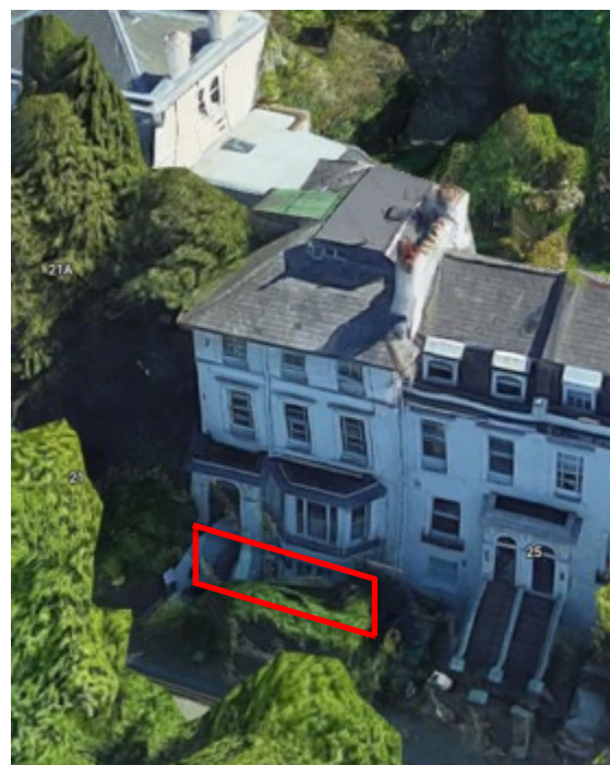
Aerial view to the street elevation
