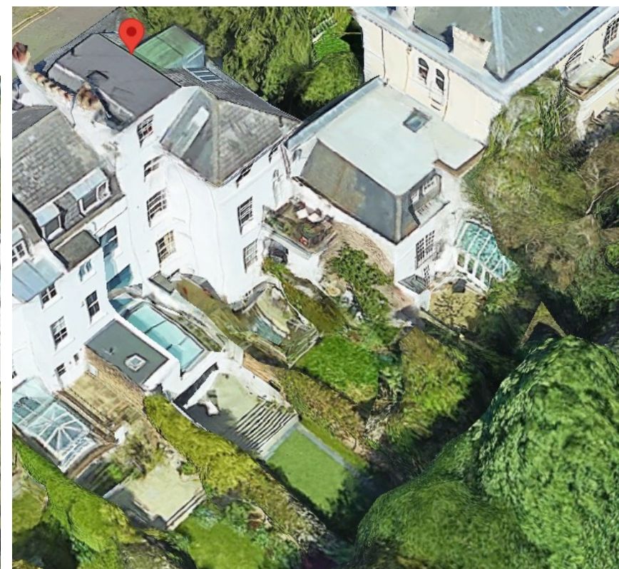
Aerial view to the side rear elevation
