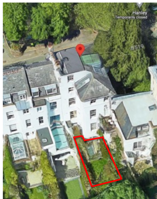
Aerial view to the rear elevation
