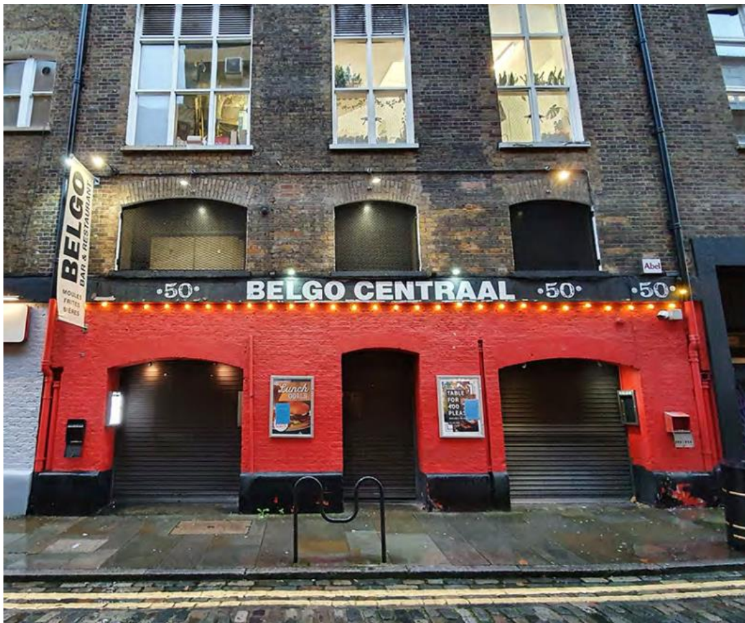
Photo 1 (above): Existing elevation fronting Earlham Street
