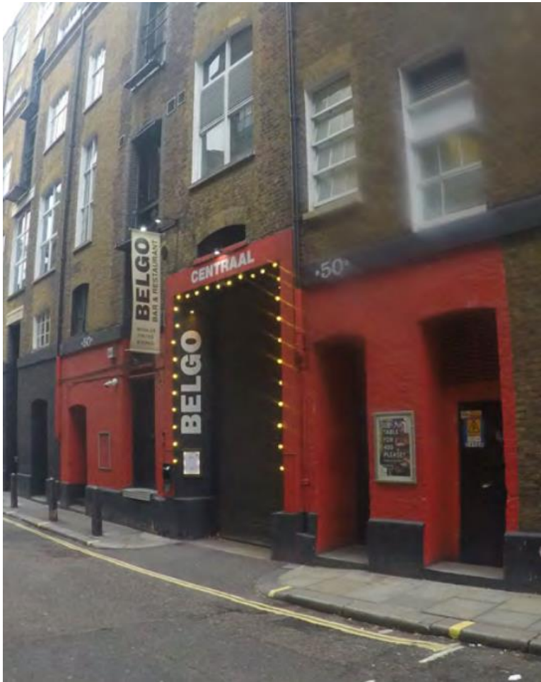
Photo 3 (above): Existing elevation fronting Shelton Street
