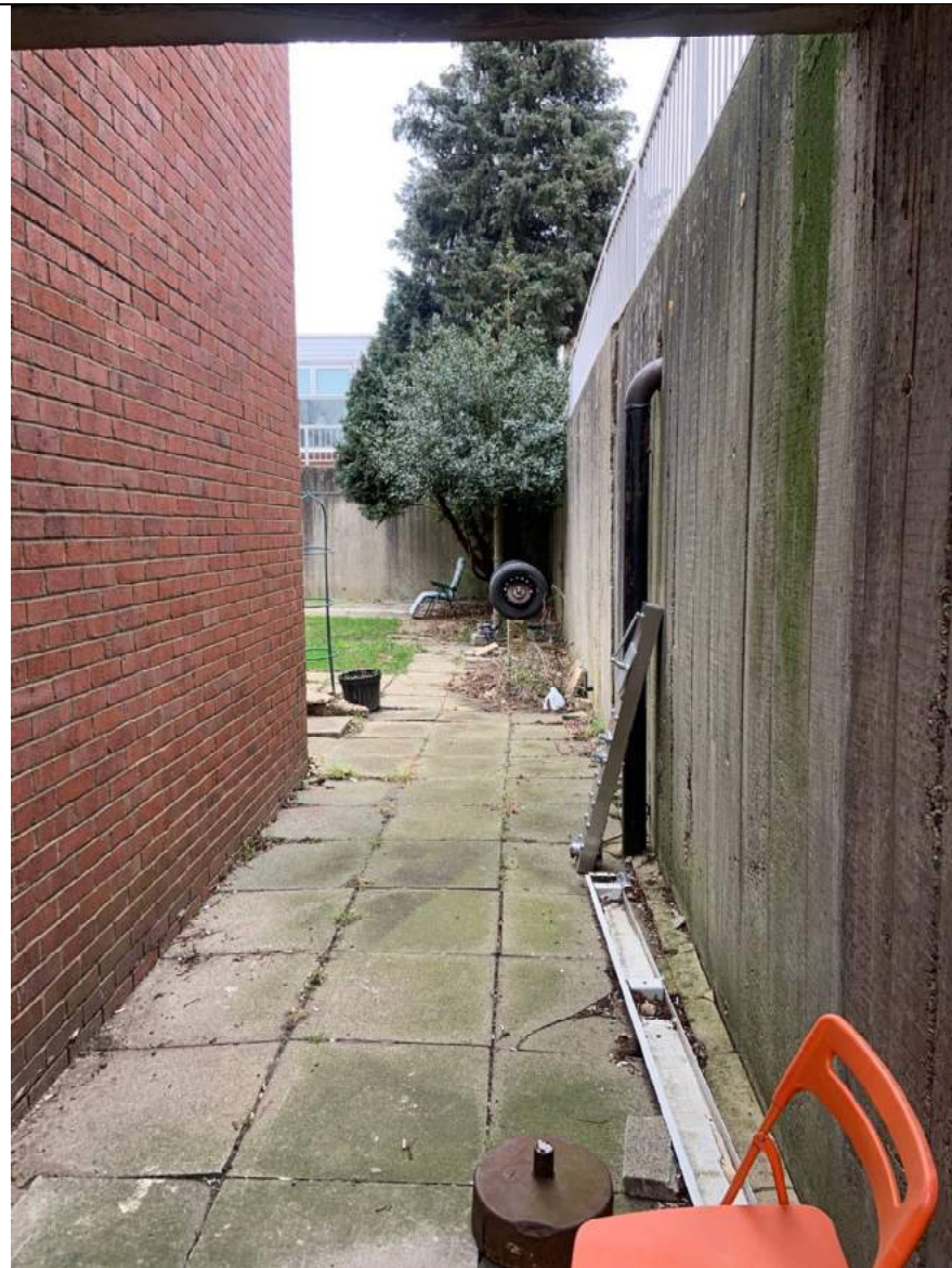
Photo 4 – Retaining wall along southern boundary.
