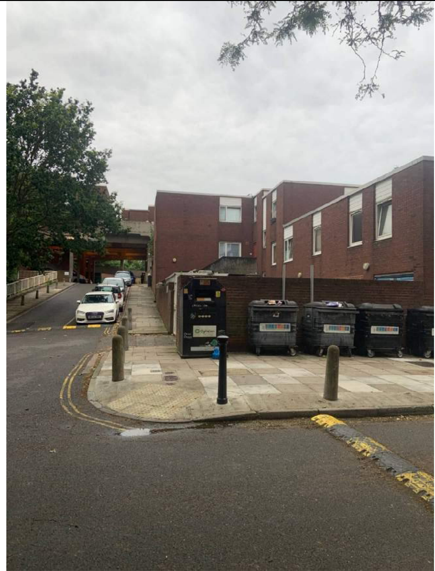
Photo 2 – View south along eastern side of site.
