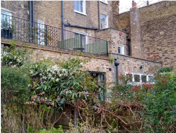
Existing extensions at 22 and 21 Steele's Road
