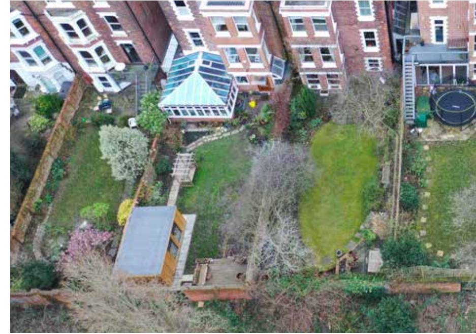
↑ Rear of No.17, showing large conservatory extension and alterations to the bay window at ground floor.
