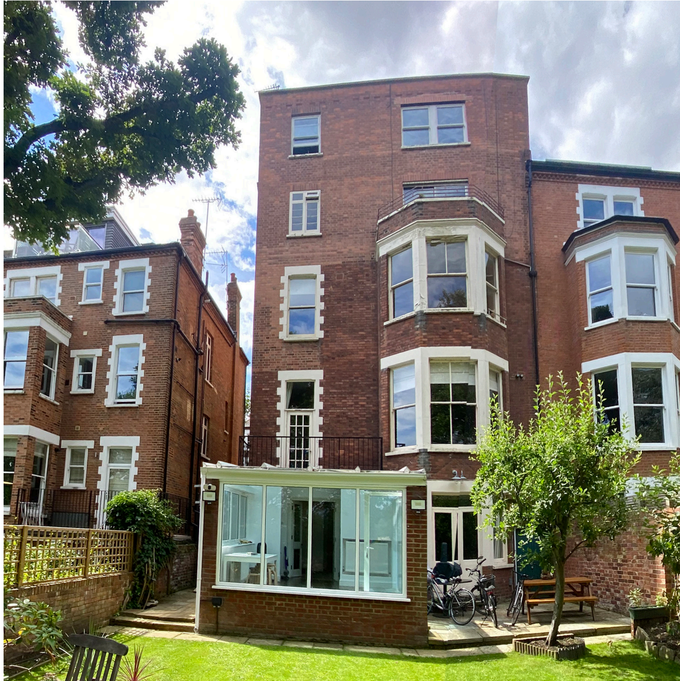
↑ Existing rear conservatory extension with UPVC glazing
